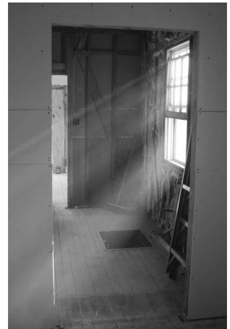
There's beauty even in drywall dust
